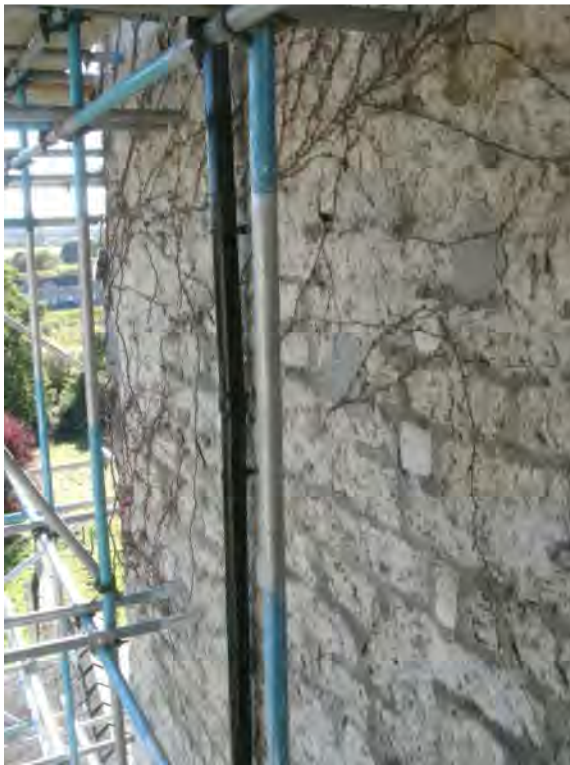
lower east wall of same
