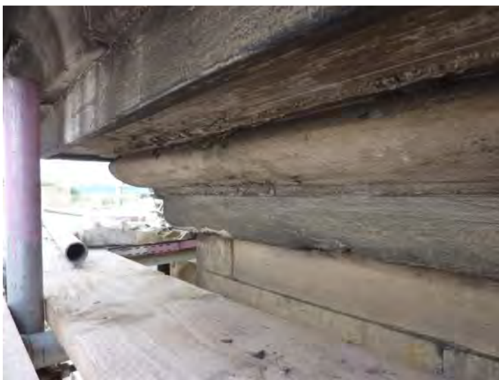
lower part of cornice
