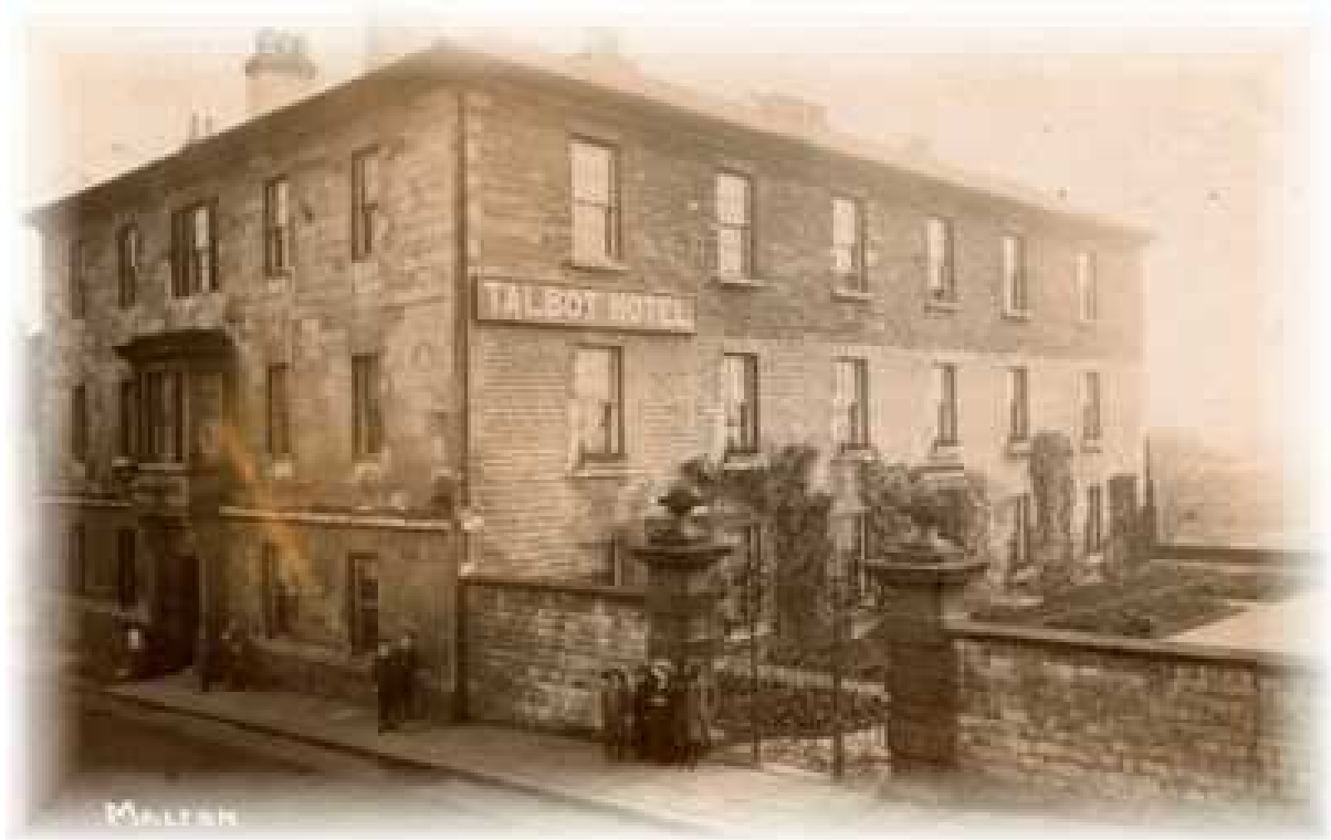
Early 20thC. Stone gate piers and railings moved to garden of Eden House, where they remain. Note different tone and character of oolitic limestone raising of west elevation
